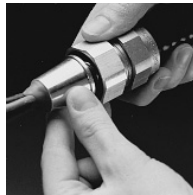
4. Slide armor stop insert over conductor and sealing compound, then back against armor. Pack remaining sealing compound.
